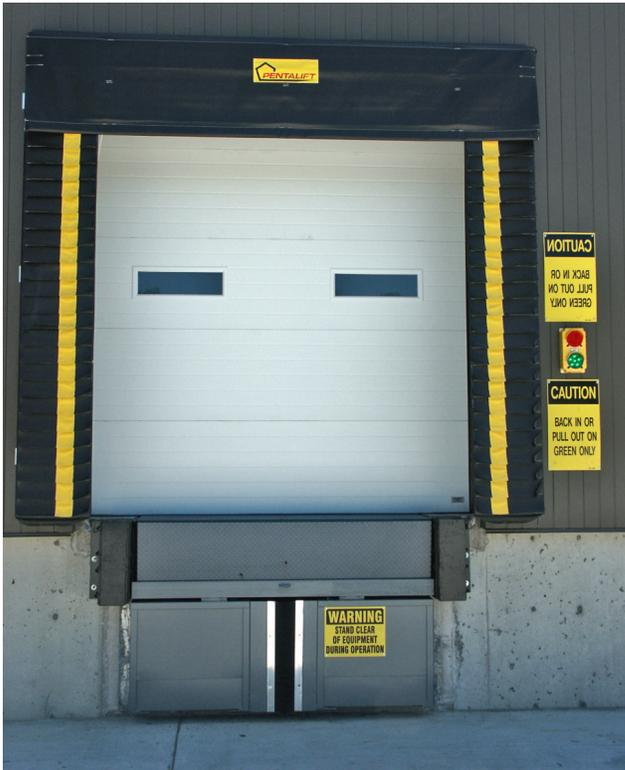
Ultrahook UHR40 is shown in the stored position ready to accept the trailer. All of the restraint components are protected under the dock leveler, away from snow, ice and debris. The installation provides a "clean" appearance.
